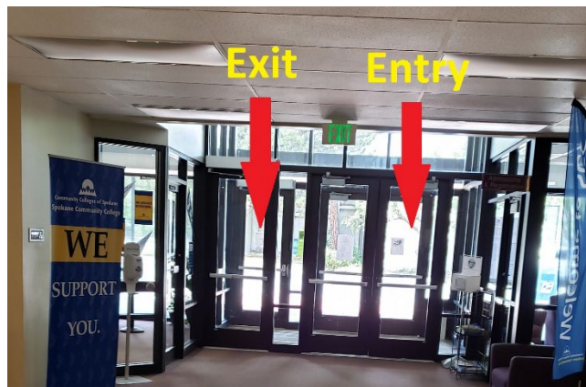
Picture 5- Building 15 Main Entrance Door
